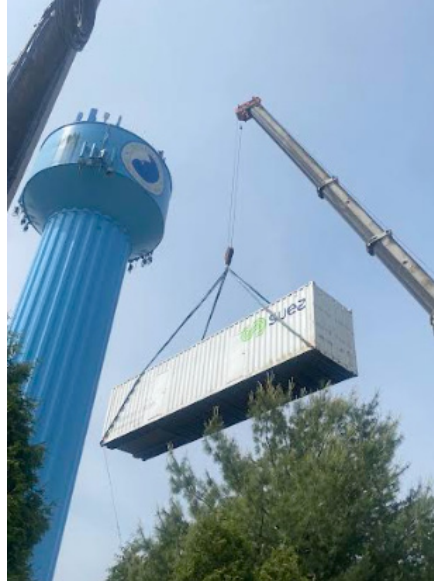
Removal of temporary PFNA system from Warren Avenue Water Treatment Facility.
